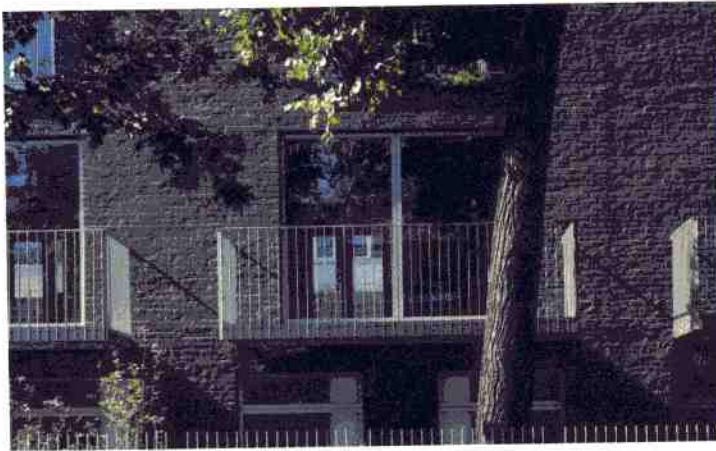
Vassall Road Housing, London
