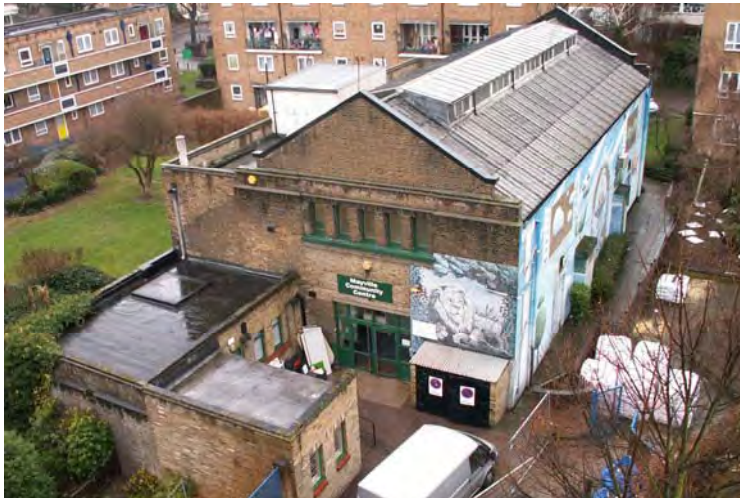
Figure 1-1 The Mayville/Mildmay Community Centre before refurbishment
