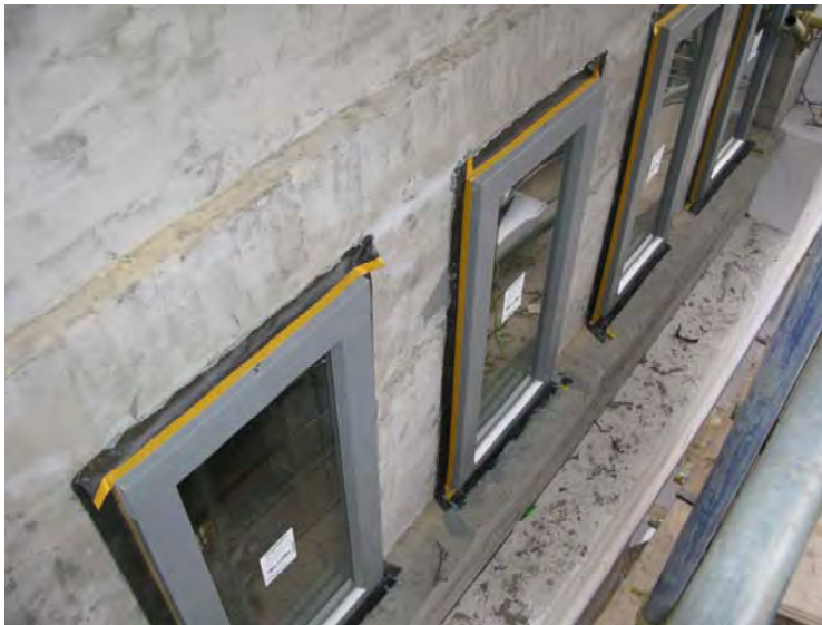
Figure 2-12 Location of windows into wall build-up
