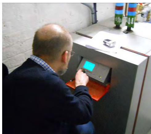
Figure 3-11 GSHP control display
