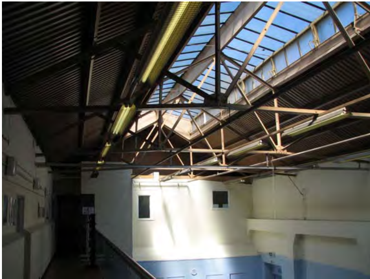
Figure 2-1 Interior view showing the main hall before the retrofit
