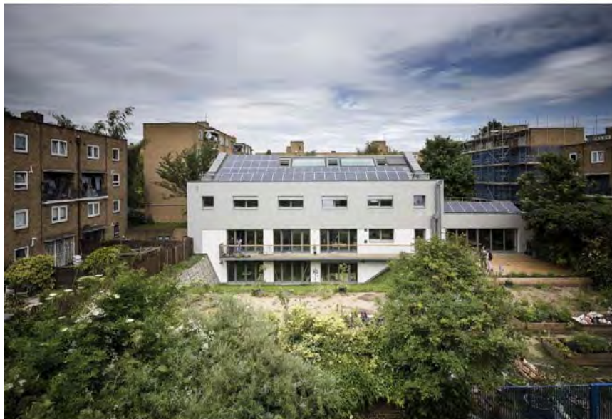
Figure 1-2 The Mildmay Centre after refurbishment
