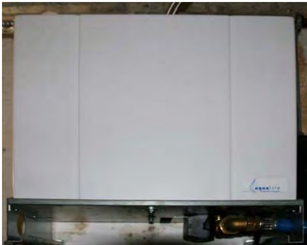
Figure 5-9 Aqualite rainwater harvesting pump
