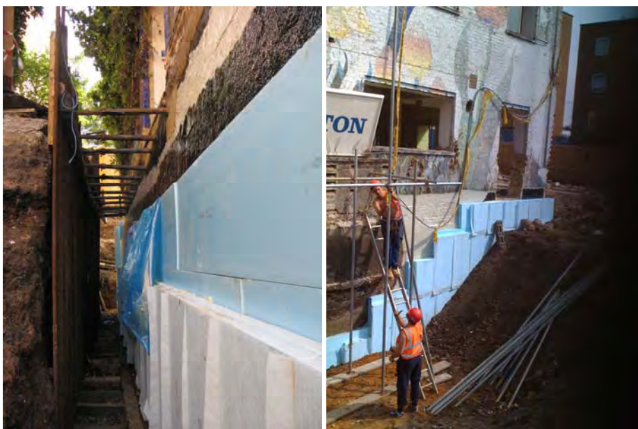
Figure 2-5 Insulation at basement level
