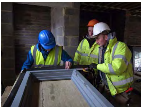
Figure 4-1 Window airtightness taping – training on site
