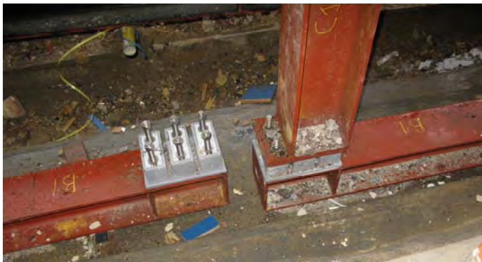
Figure 2-7 Steel posts with thermally broken connections (by Schöck) for the basement openings
