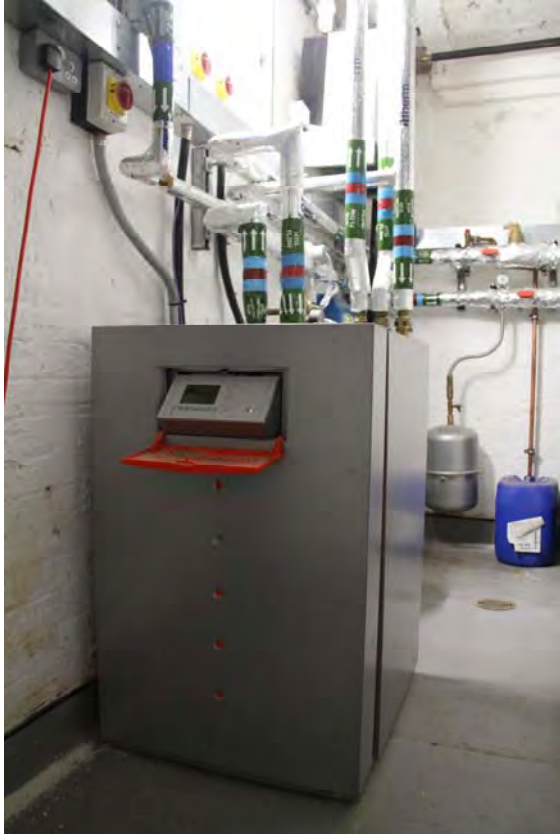
Figure 3-8 Ground source heat pump (GSHP)
