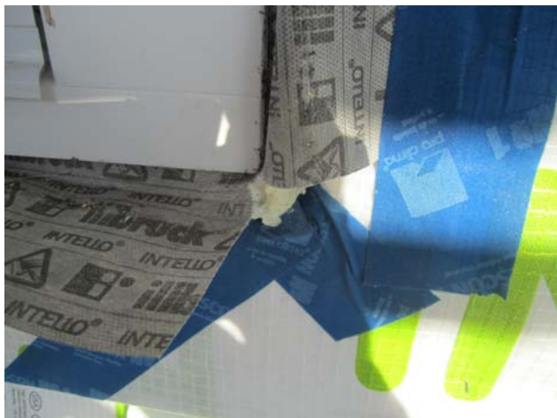
Incorrectly installed
