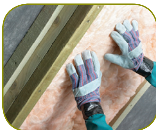
Internal wall insulation being fitted
