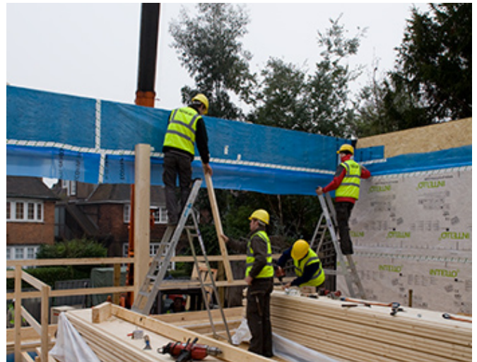
Air tightness Intello membrane and tapes exposed
