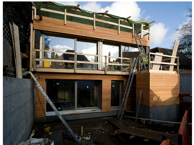
View of the front of the house under construction
